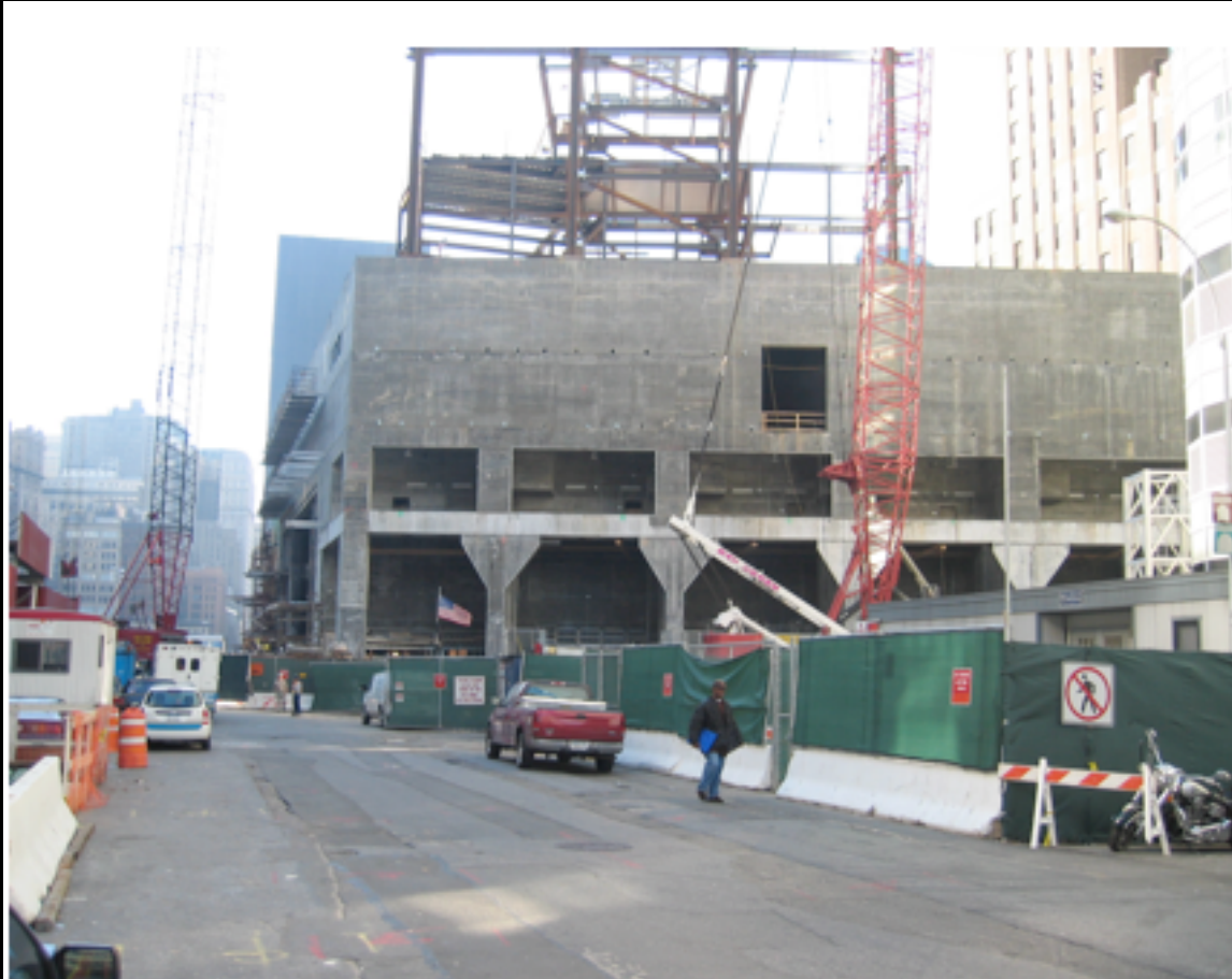
Fig 5.6 The entire base section of 7, World Trade Center -- one of the skyscrapers constructed on the site of the destroyed World Trade Center -- consists of a blast-proof concrete which was later hidden by a colourfully lit screen
